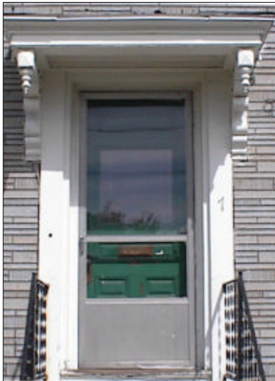
Left: Single wood paneled doors like this one are found throughout the district. The brackets supporting the roof, or pediment, over the doorway are also a common feature.
