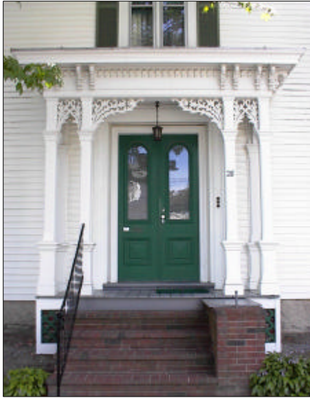
Left: This porch has several key Italianate elements, including paired brackets, double doors with arched glass panels, and paired porch columns.
