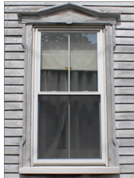
Lower Left: The bold profile on the hood and surround of this window represent another common Italianate characteristic.
