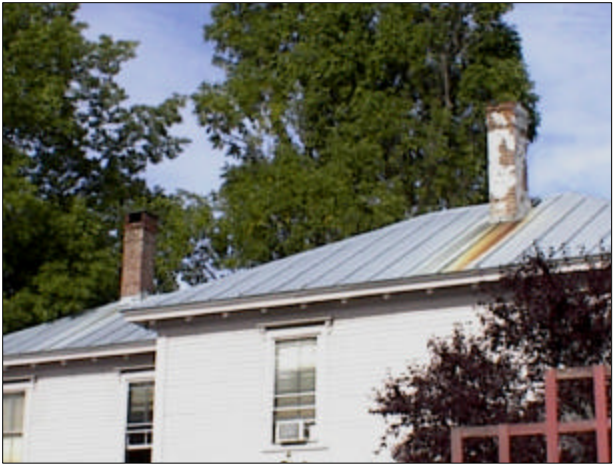
Above: Hipped roof with a standing seam metal roof. The width between seams establishes a strong pattern, which contributes to the character of the building. Typically, metal roofs in the district are aluminum or pewter colored, as opposed to bright colors.
