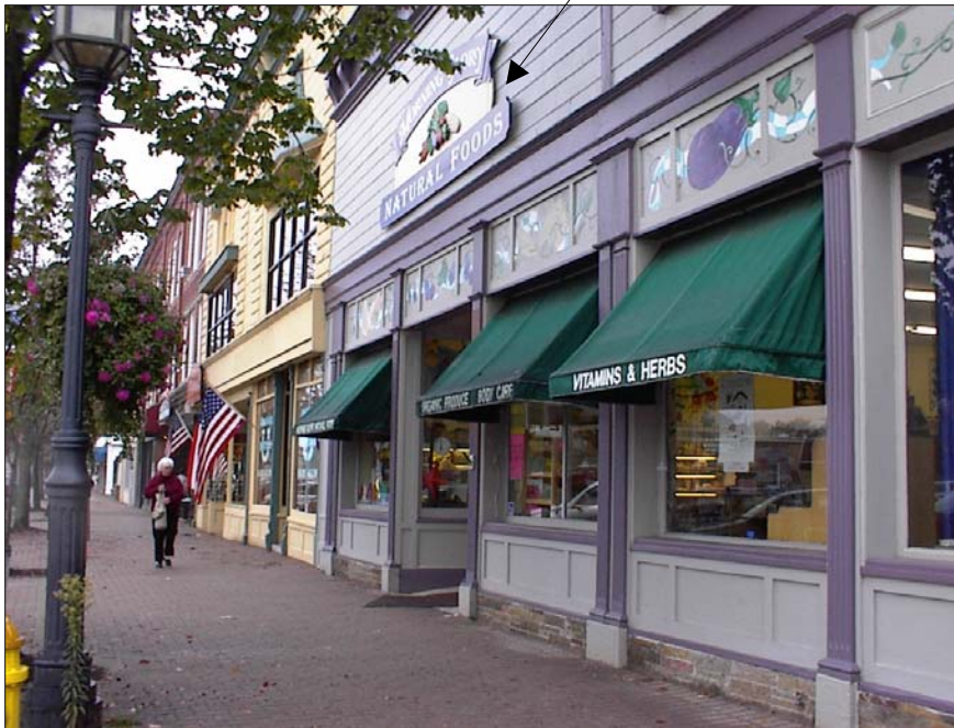
Flush mounted sign.
