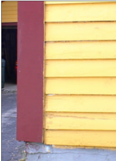
Left: Simple corner board and wood clapboards.
